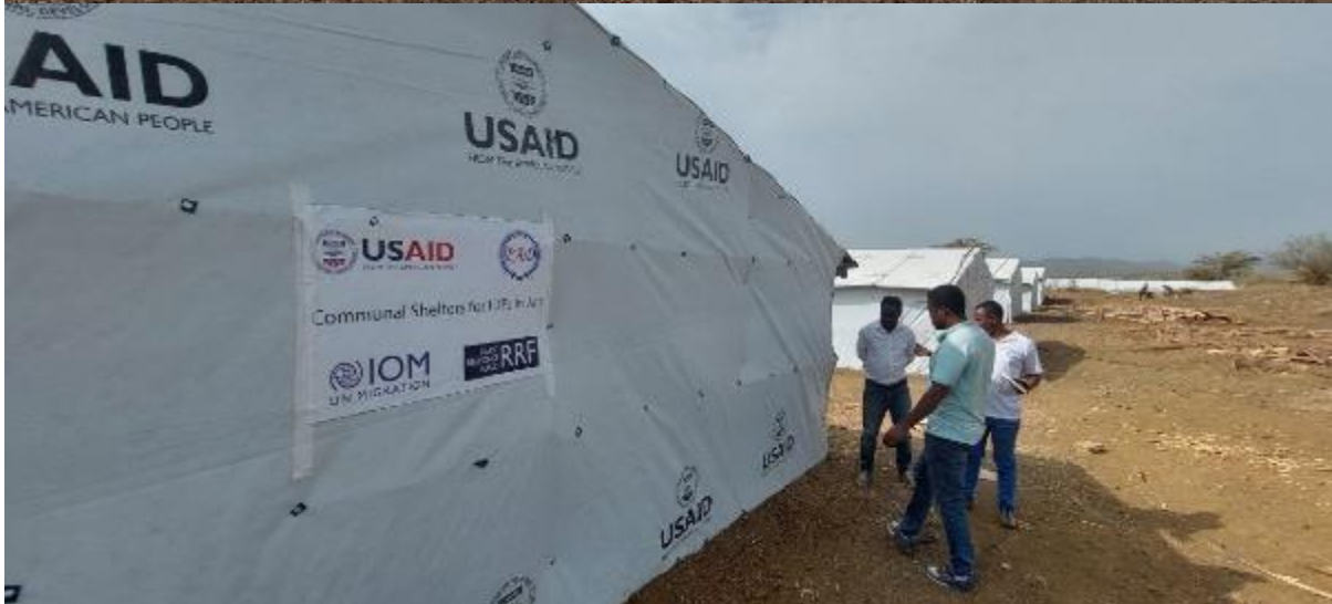
IDPs Shelter Construction
